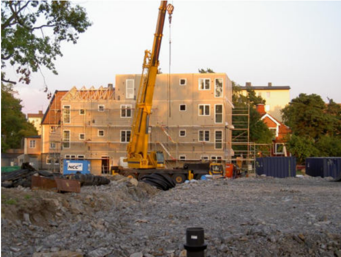
Volume elements; typical sizes: 4 500 (w) x 3 000 (h) x 13 500 (l)
